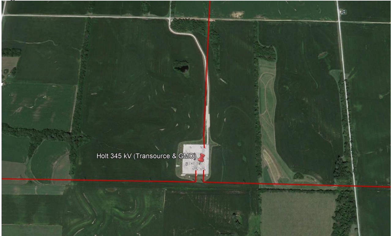
Figure 29 – Holt 345kV Substation
