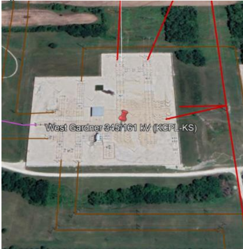
Figure 24 – West Gardner 345kV substation
